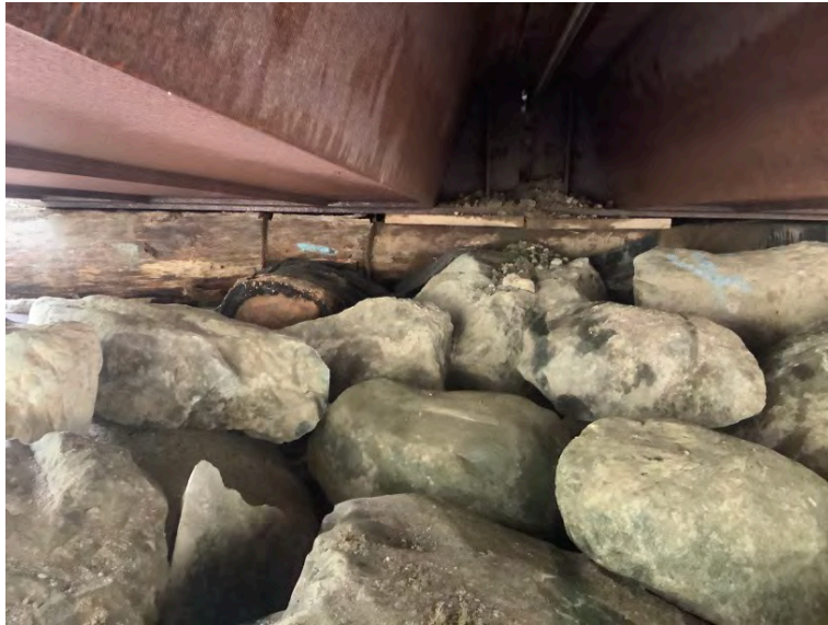
Right Bank Abutment when facing downstream
