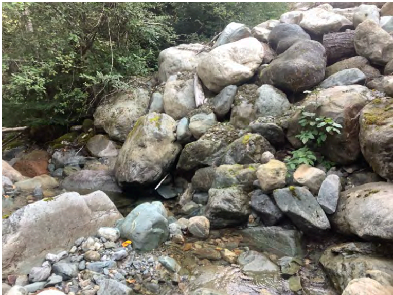
Right Bank Abutment when facing downstream
